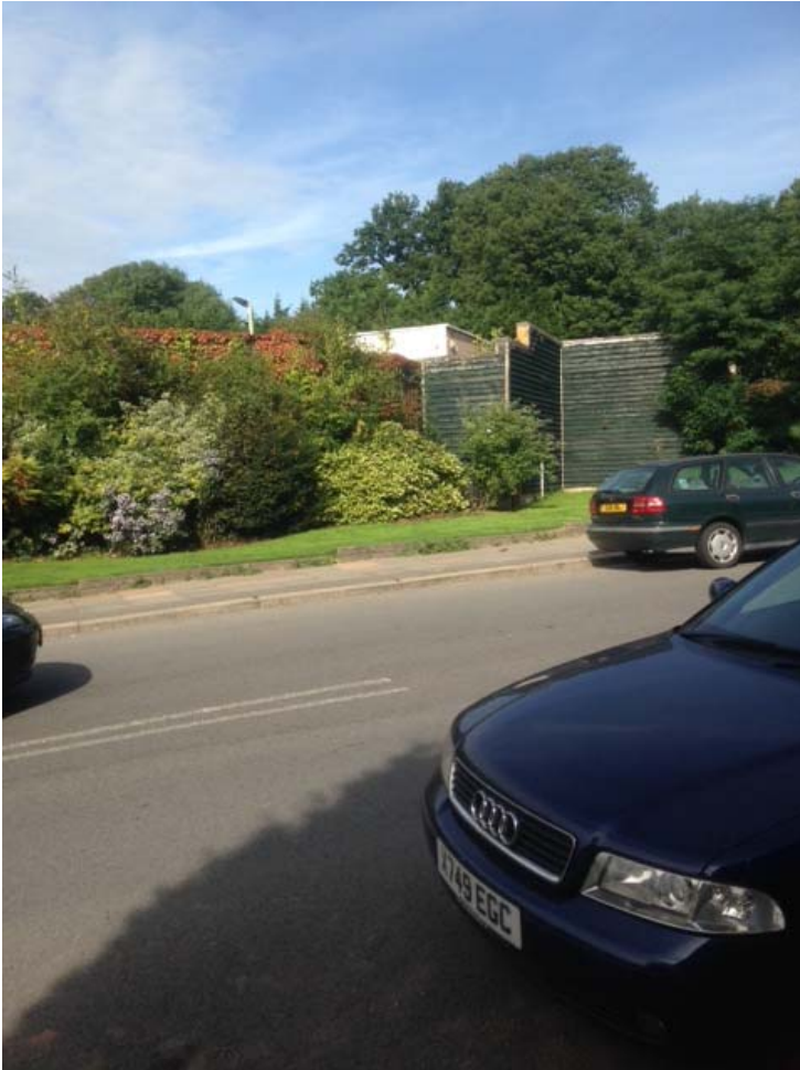
View of the damage caused to the existing building
